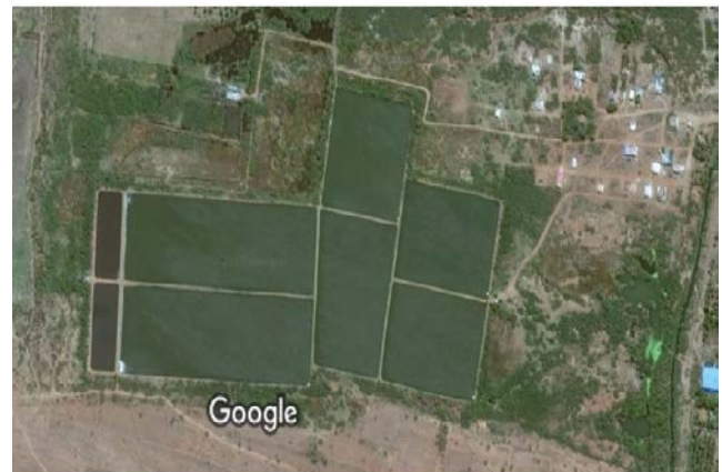
Figure 5.3.2 WATER TRETMENT SITE
